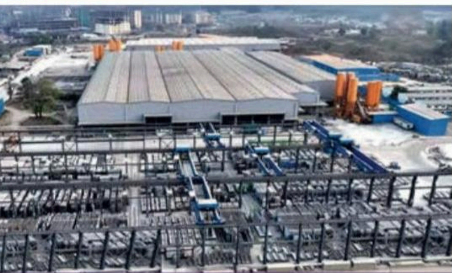
CASL Precast Plant at Suraksha City, Vasai, Mumbai
